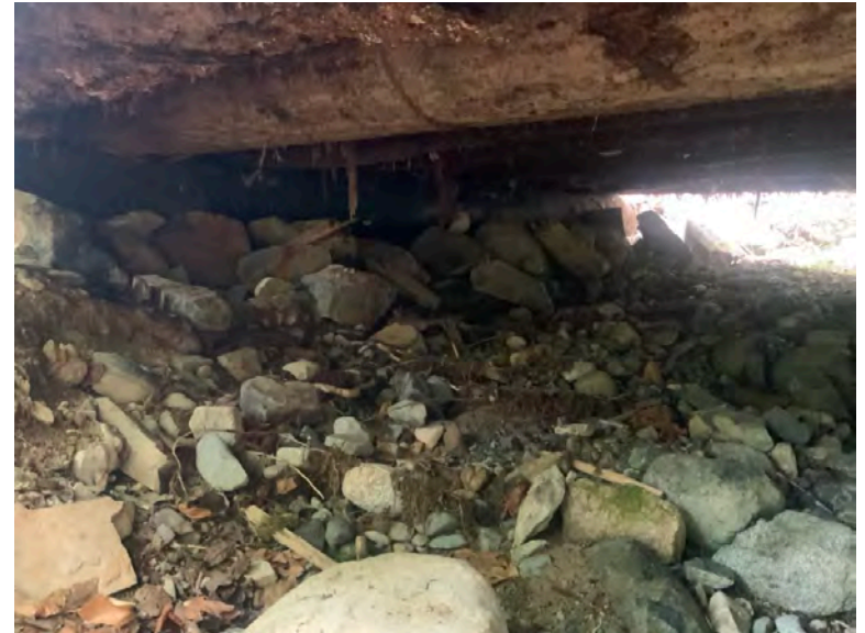
Right Bank Abutment when facing downstream
