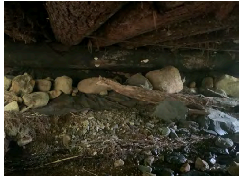
Left Bank Abutment when facing downstream
